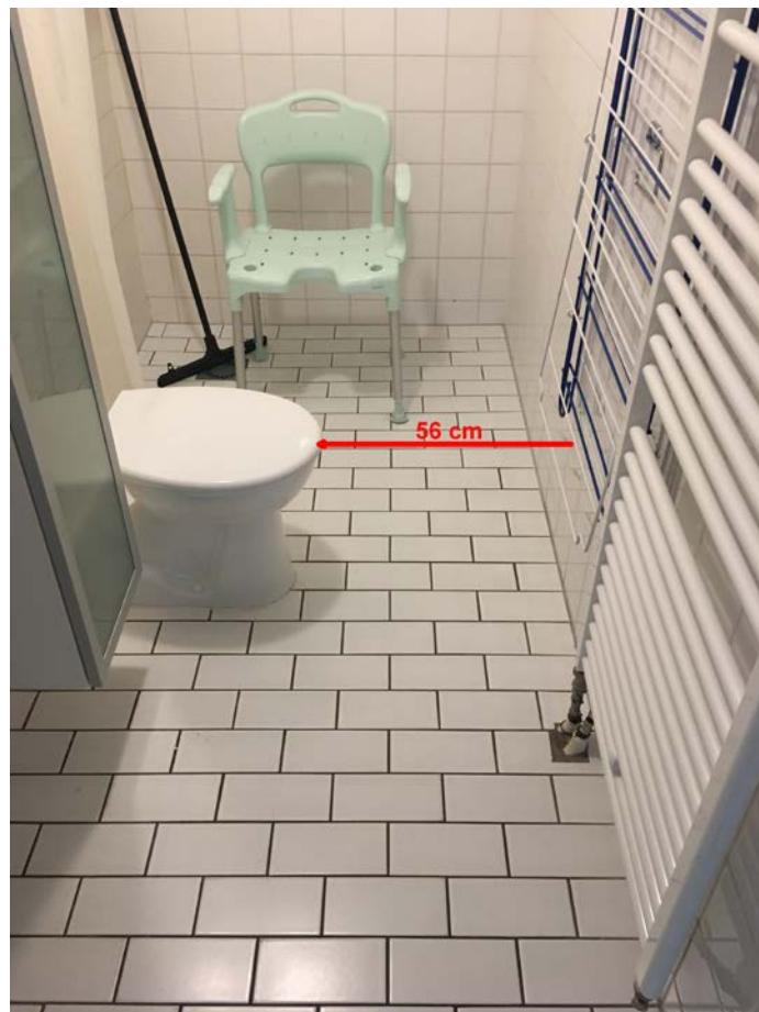
Bungalow 510 bathroom (not WC accessible)
